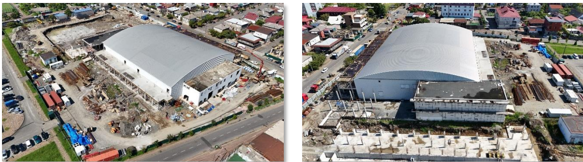
Figure 4: Batumi Ice Arena; Ice Arena construction site photo
