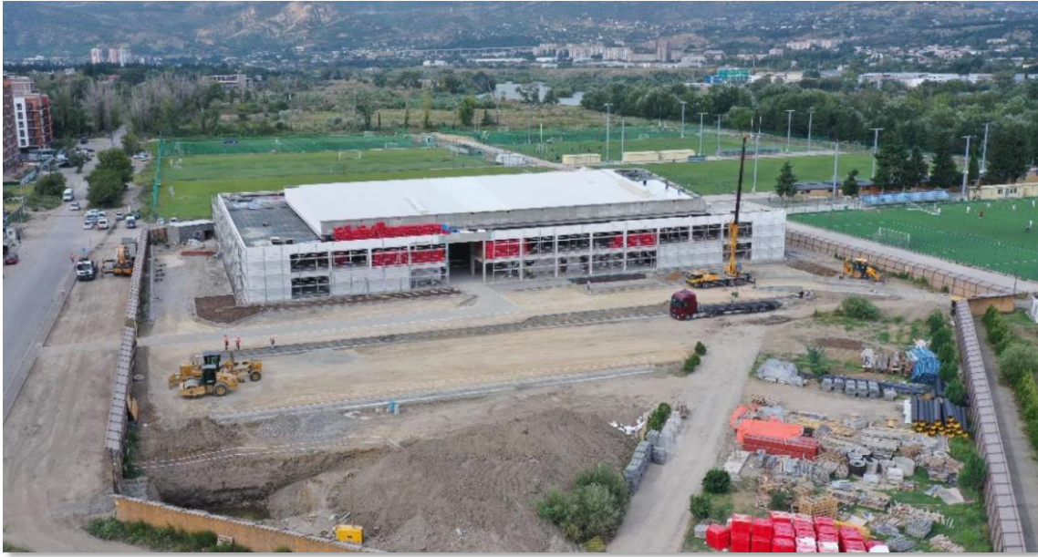
Figure 4: Tbilisi Ice Arena; Ice Arena construction site photo
