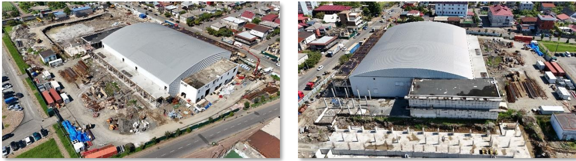
Figure 4: Batumi Ice Arena; Ice Arena construction site photo
